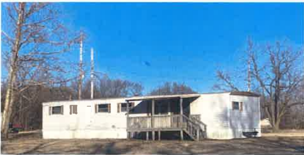
▲ Figure B.2. Mobile Home in Sound Condition
