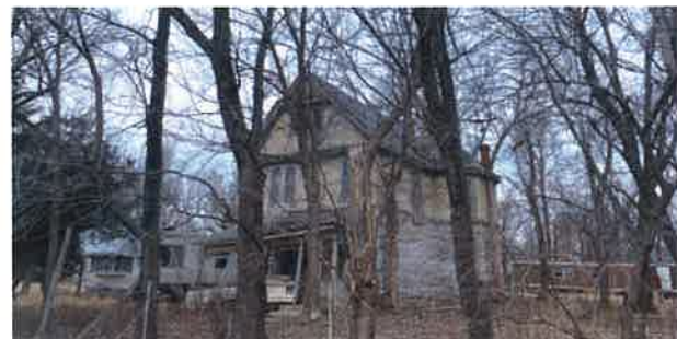
▲ Figure B.6. Single-Family Home in Dilapidated Condition
