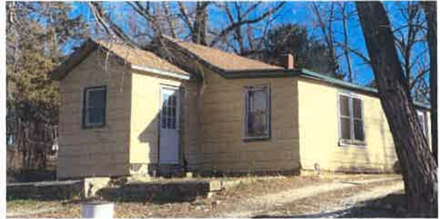
▲ Figure B.4. Single-Family Home Needing Moderate Rehabilitation
