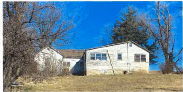
▲ Figure B.5. Single-Family Home Needing Substantial Rehabilitation
